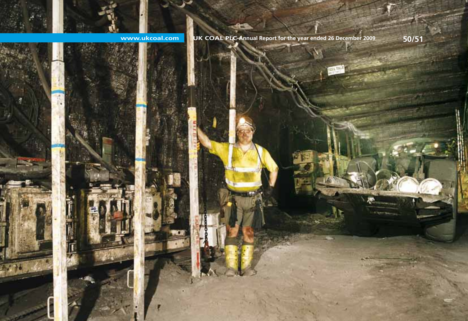
PICTURED: The steel sentry safety system designed to prevent equipment being damaged by passing vehicles taking materials underground.
